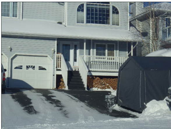
Inadequate Combustible Storage
