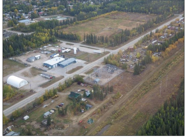
Fort Smith Substation and Powerplant
