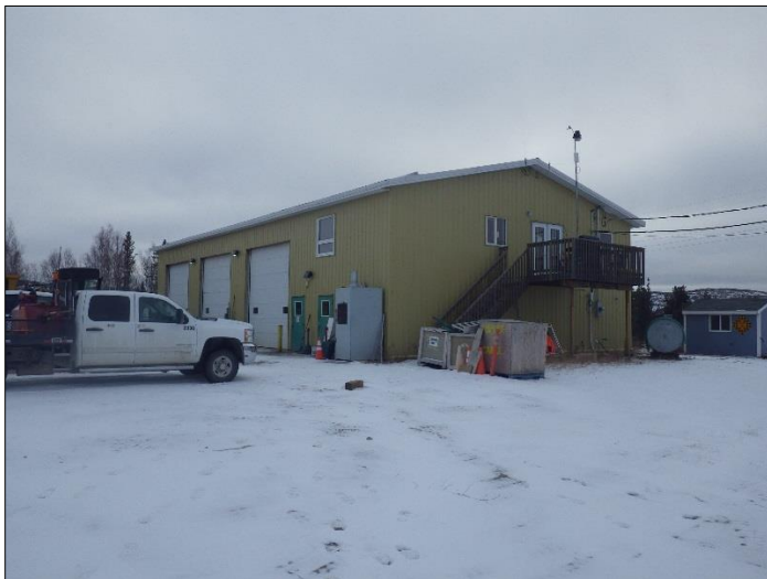
Snare Airstrip – Wooden Steps/Deck & Combustible Materials
