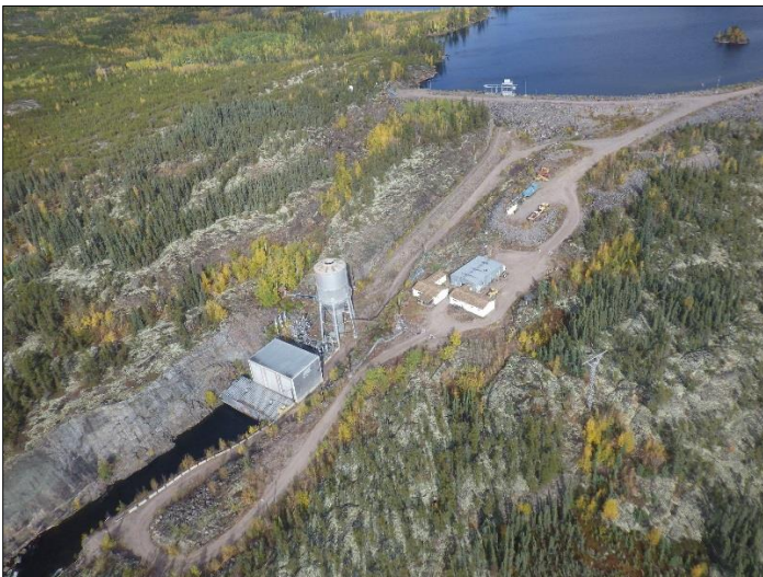
Powerplant, Sump Shack, & Camp – Minimal Threat
