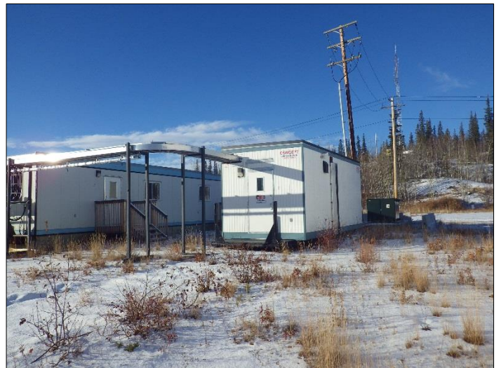
Equipment Storage & Camp – Inadequate Zone 1
