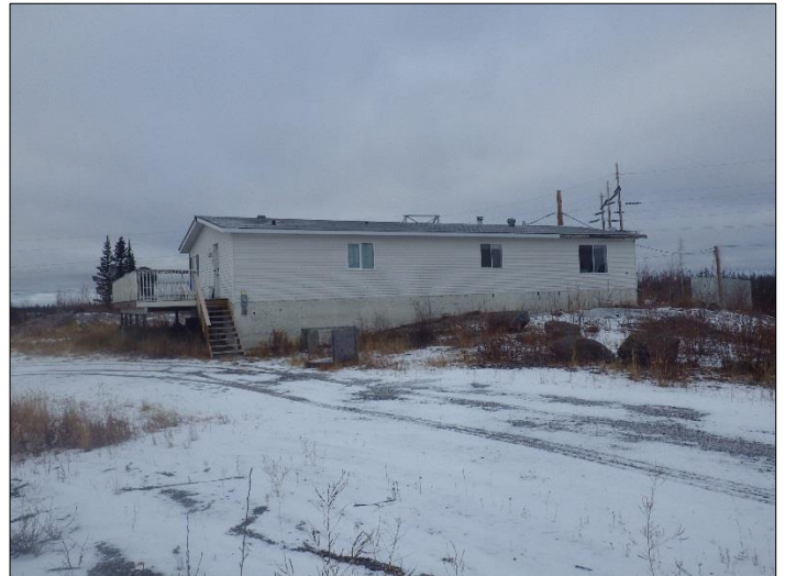
Snare Cascade Staff House – Inadequate Zone 1 Clearance
