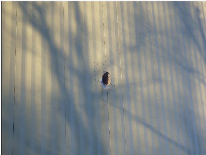
Headgate – Patch Hole in East-Side of Building
