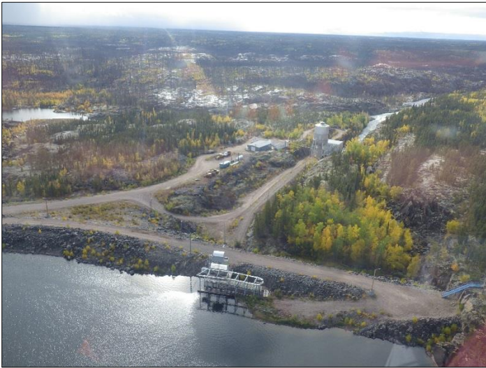
Headworks – Minimal Threat
