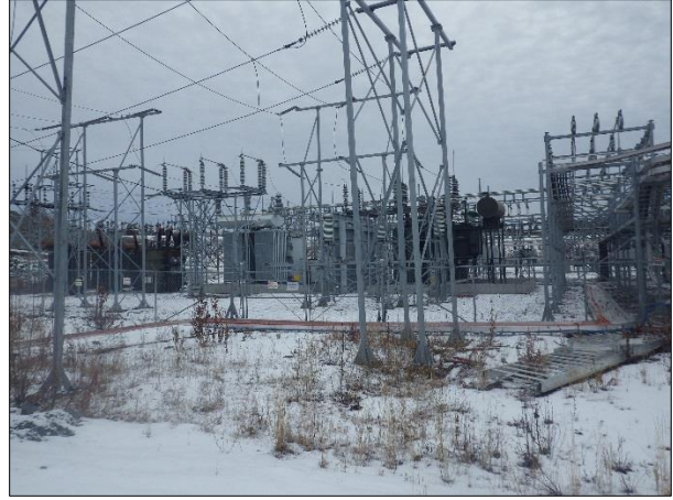
Adequate Zone 1-2 Clearance
