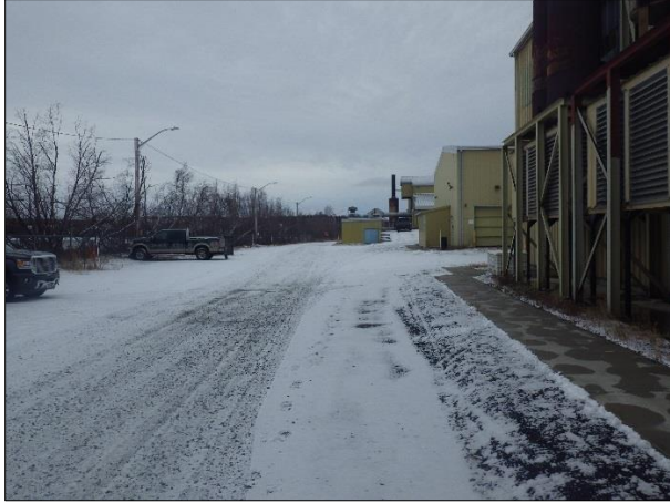
Adequate Zone 1-2 Clearance
