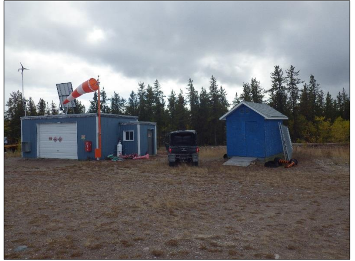
Airstrip & Buildings – Inadequate Zone 1 Clearance
