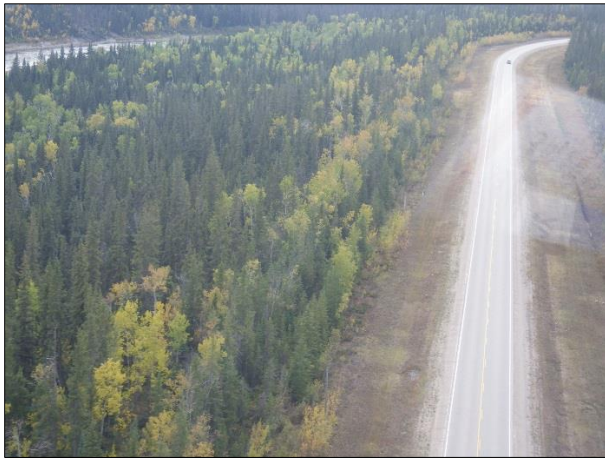
Wooden Poles – Pine Point to Hay River
