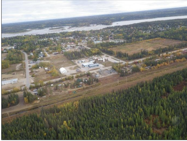
Fort Smith Substation and Powerplant
