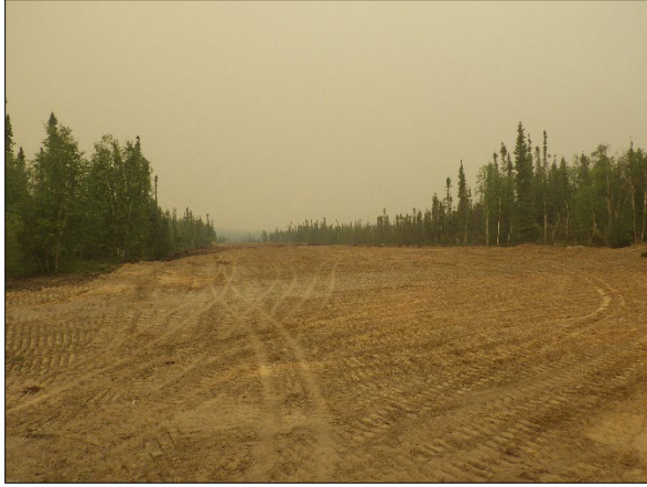
After Mechanical-Clearing (East Fireguard)
