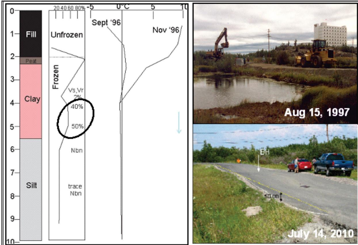
Figure 35. A borehole drilled in 1997 shows frozen ice-rich clays with percent (%) visible ice beneath the access road to the Prince of Wales Heritage Centre. The road was insulated and paved in 1997 and by 2010 had settled by up to 50 cm. Driving the road today illustrates that settlement continues and that ongoing maintenance will be required.
