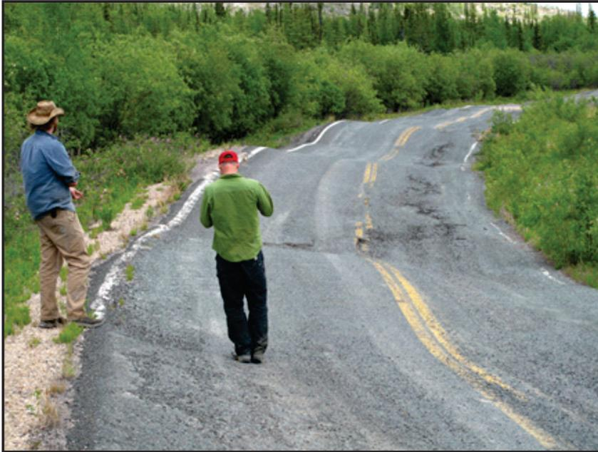
Figure 29. Abandoned section of Highway 4, east of Yellowknife. The paved road surface has continued to settle due to permafrost thaw after it was abandoned in 1999.
