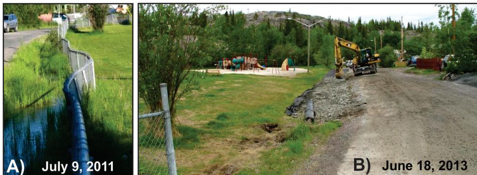
Figure 39. Fritz Thiel Park. A) The fence line indicates subsidence and surface movement. B) Infilling of subsided terrain and repair of the road embankment and fence on Stout Road.
