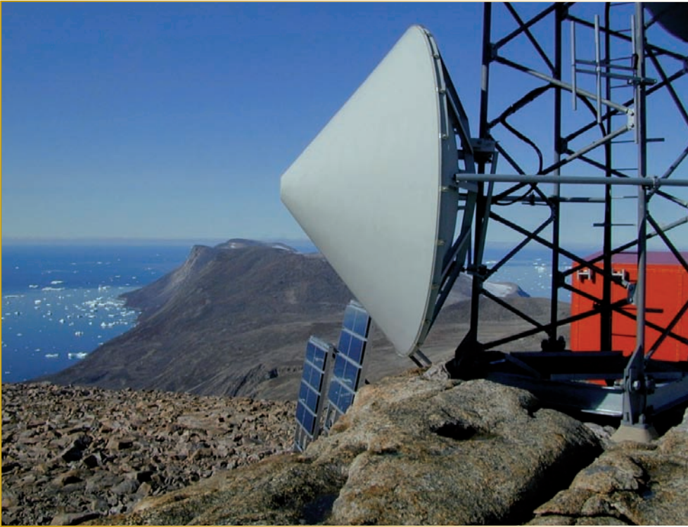
Hill-top relay station in West Greenland, with solar panels (photo: Tele Greenland Ltd.).
