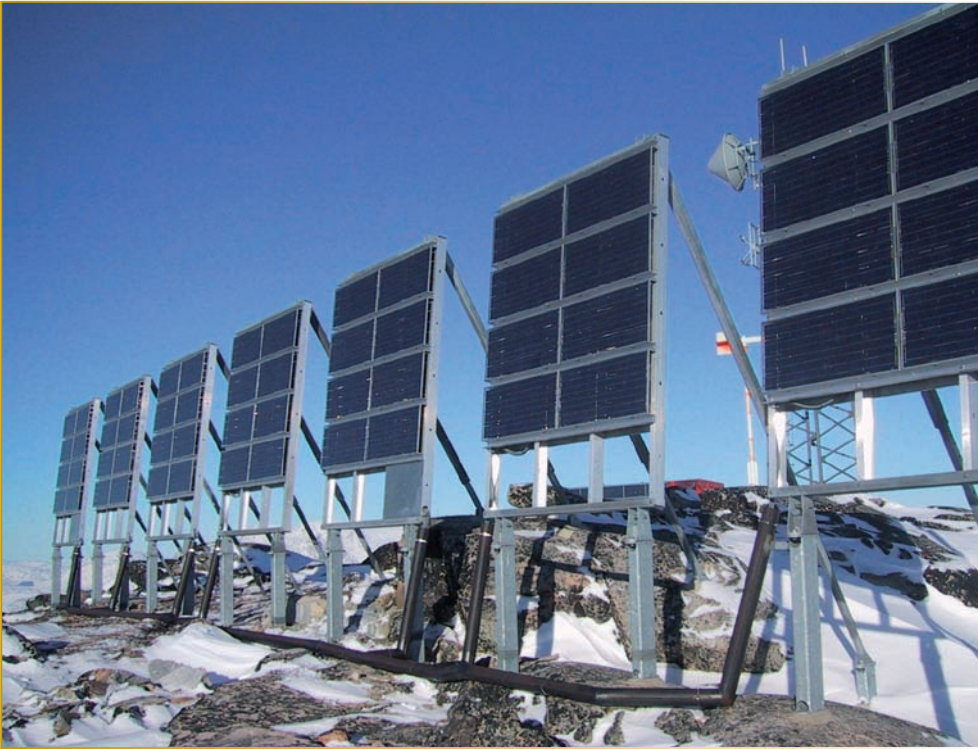
Solar panels at a hill-top relay station in West Greenland (photo: Tele Greenland Ltd.).
