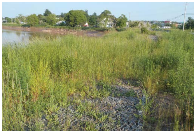
FIGURE 24: Hybrid living shoreline on the Shubenacadie River, Bay of Fundy, NS, illustrating gabion basket planted with marsh vegetation to reduce erosion scour. Photo courtesy of V. Leys, August 2015.
