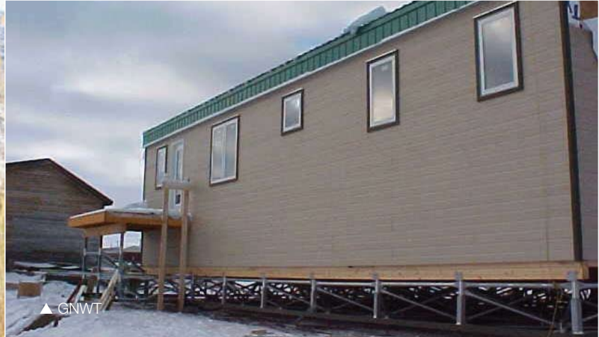
▲ Foundations that distribute weight and absorb stress limit problems caused by ground movement – Triodetic Building Products Ltd.
