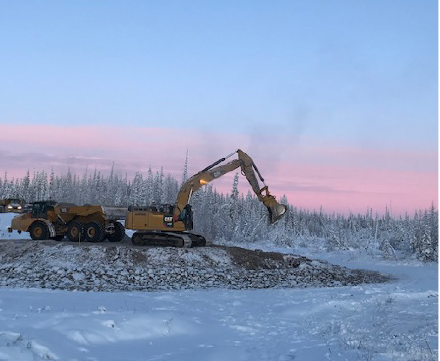
Embankment Construction, NWT
