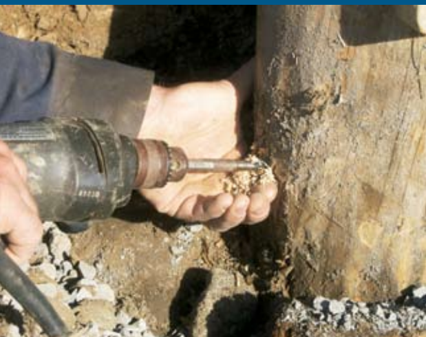
Sampling of pile interior allows detailed diagnosis of wood rot progress in a lab.
