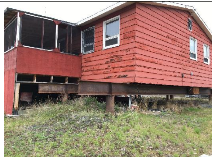
Southeast corner of office building
