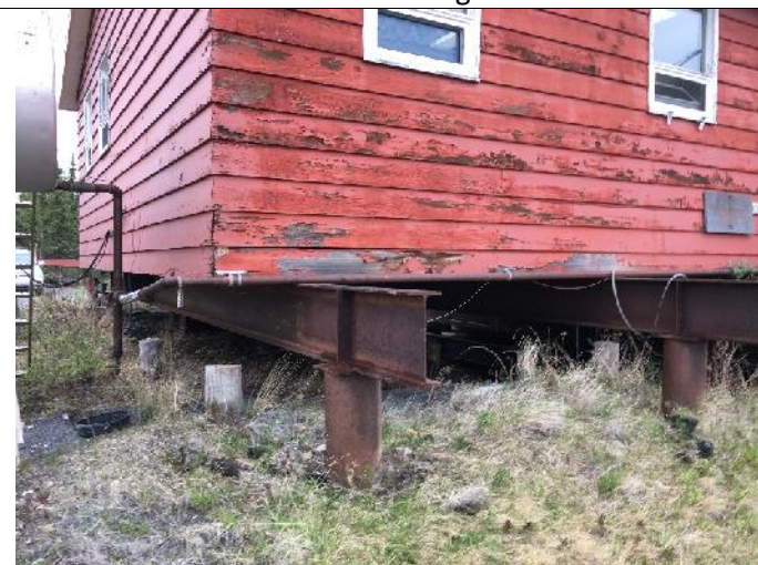
Southwest corner of building. Cutoff wood piles visible
