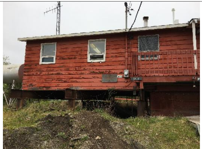
Southwest corner of office building
