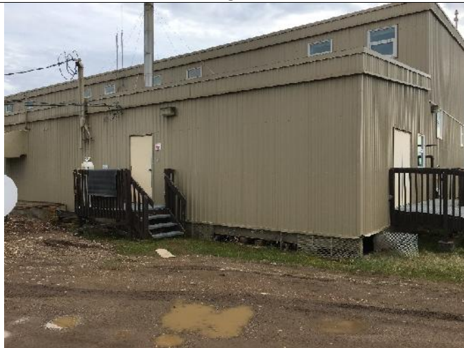
North side (back) of building
