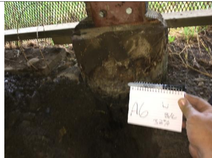
A7 – Incorrectly labelled as A6
