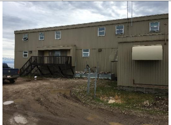
North side (back) of building
