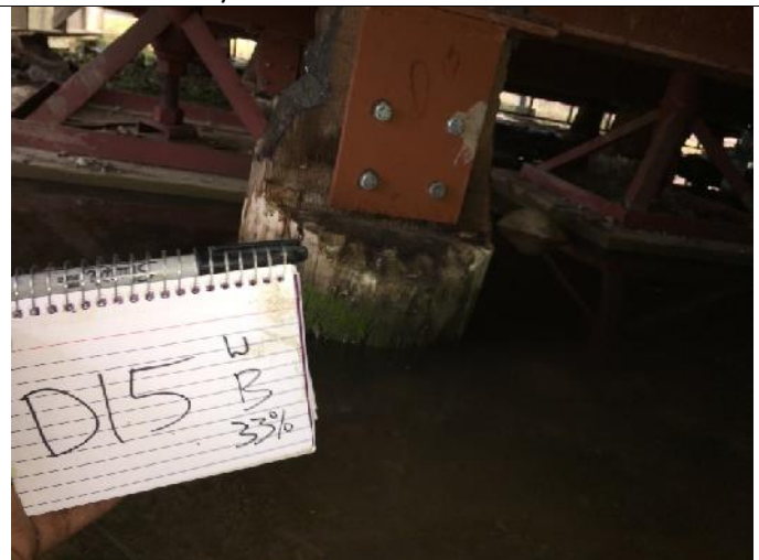
E15 – Incorrectly labelled as D15
