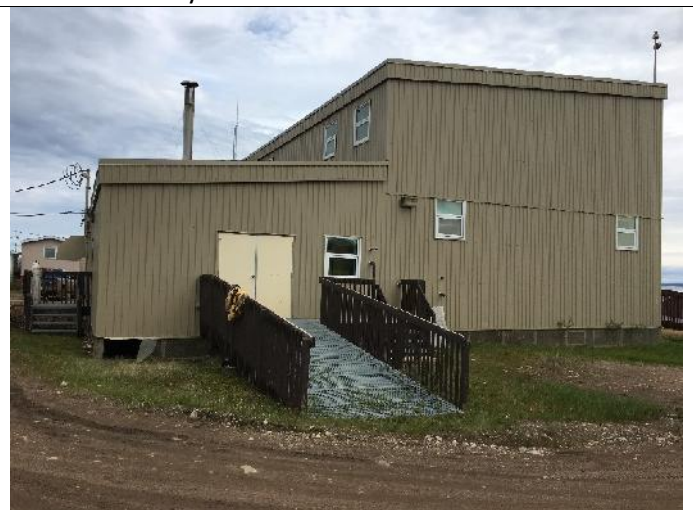
West side of building
