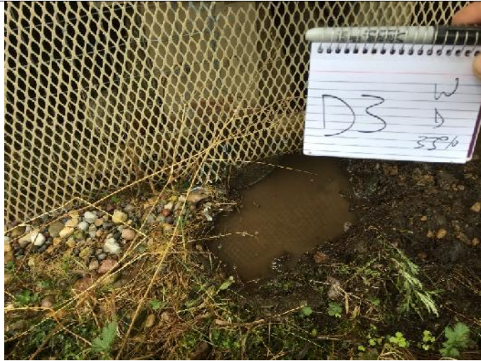
H3 – Incorrectly labelled as D3
