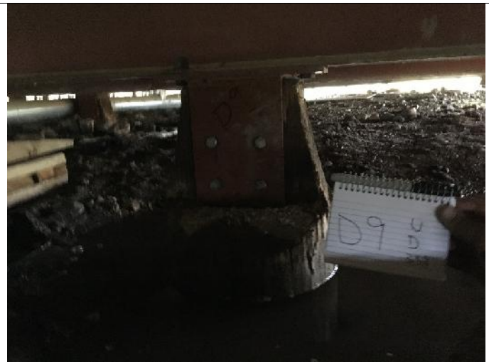
E9 – Incorrectly labelled as D9
