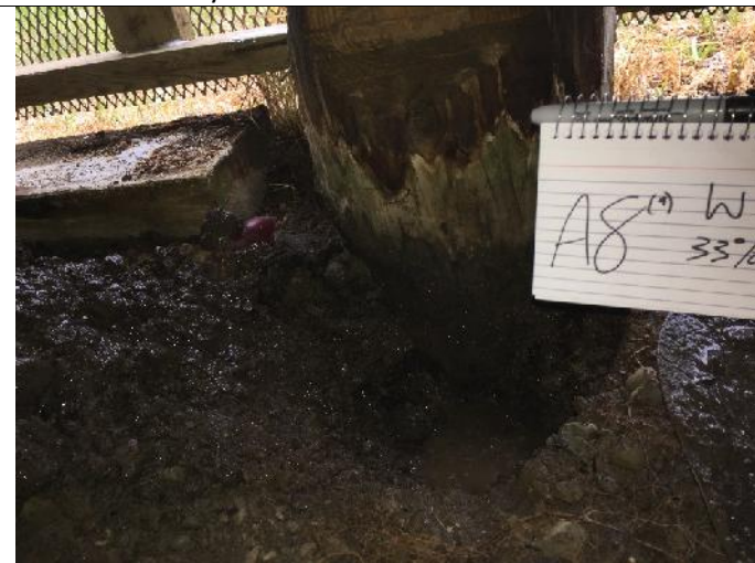
A9 – Incorrectly labelled as A8
