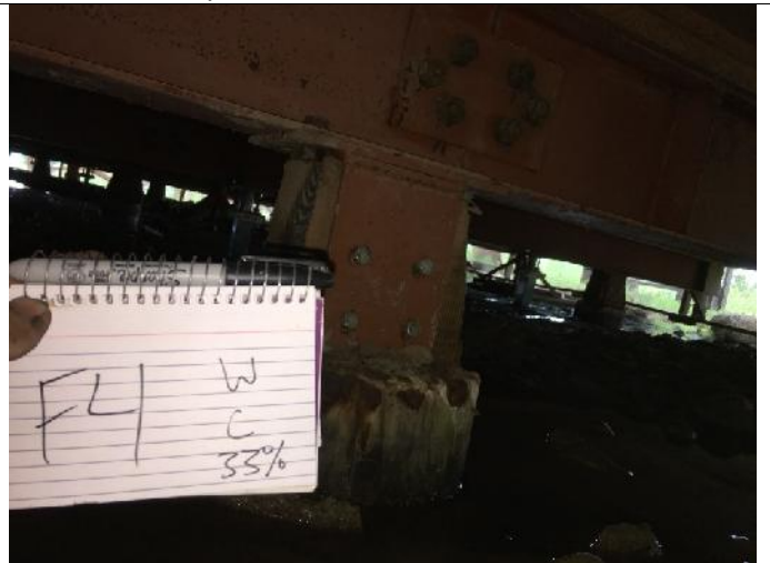
G2 – Incorrectly labelled as F4
