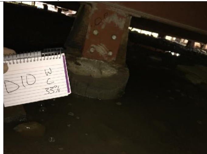
E10 – Incorrectly labelled as D10
