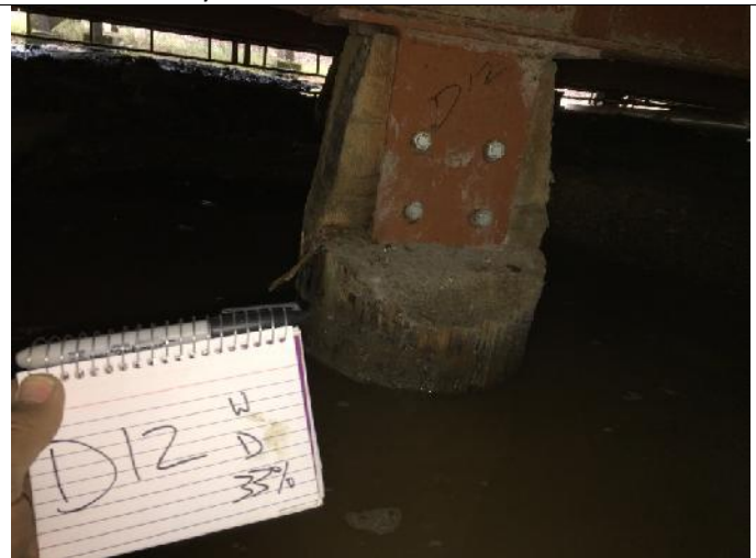
E12 – Incorrectly labelled as D12
