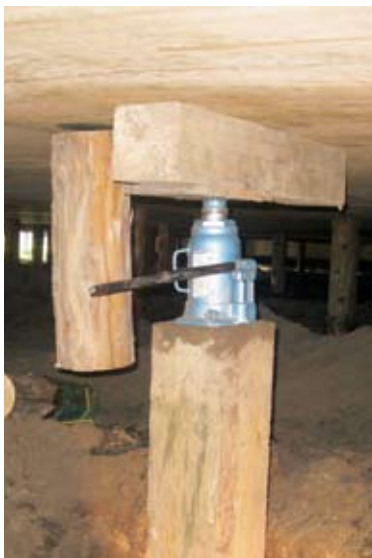
Temporary support allows new pile sections to be installed.
