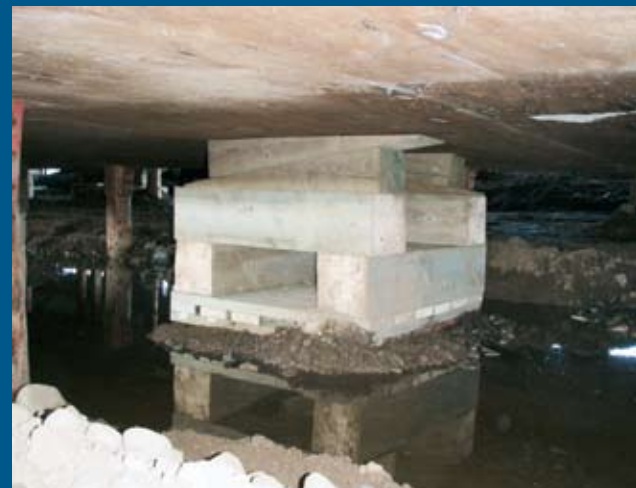
Wood crib blocking provides interim support for failed pile. Water must be drained to eliminate frost heaving.
