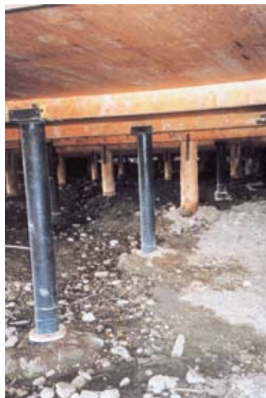
New steel posts connect solid piles below the earth to the building.
