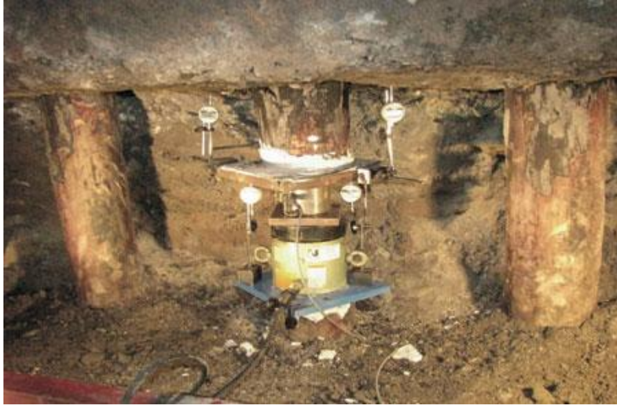
Figure 4. In-situ load testing of timber pile
