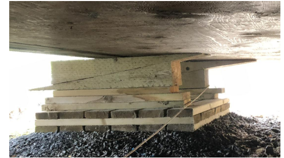
TYPICAL BLOCKING DETAIL
