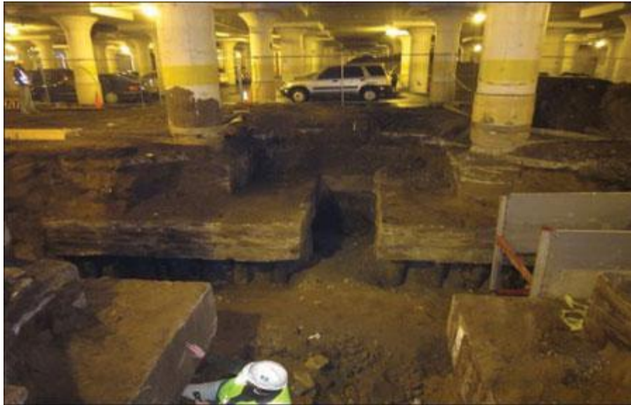
Figure 2. Overall view of track deck structure at first test pit excavation
